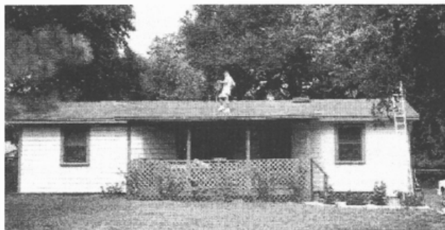
Figure 1. Photo of test site from the east.
